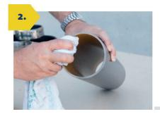
Clean the pipe surface inside and outside 3 cm wide until it is dry and free from grease and dust.
