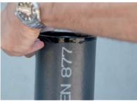
Fold **PREIS® PEP** from the inside out and firmly press to the whole circumference of the outside of the tube until the cut edge is completely covered by **PREIS® PEP.**
