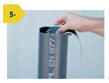
Apply **PREIS® PEP** to the inside of the cut pipe, taking care that the application is straight, so half the width (about 15 mm) extends beyond the pipe edge.
