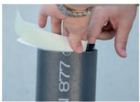
Taking care to avoid creases, press **PREIS® PEP** firmly to the inner surface and remove remaining protection.
